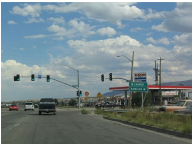
Figure 2. Intersection in Mills that was recently completed.
